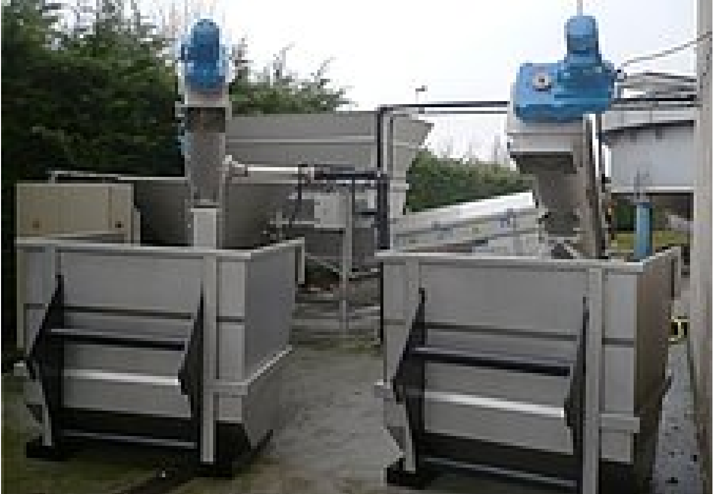
HUBER's first small grit treatment plant in France for treatment of sewer grit and road sweepings
