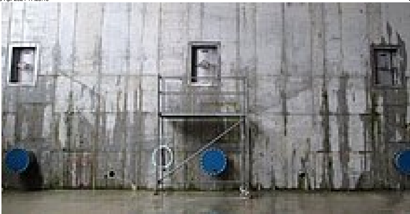
Fig. 2: The three TT7-30 pressure doors shortly after installation into the ozone reaction chambers at the Echthausen waterworks
