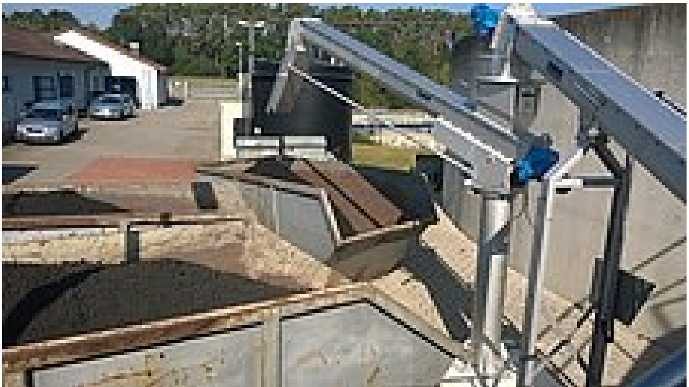
HUBER Screw Conveyor Ro8 T transporting dewatered sludge on STP Hausen. Freely rotating discharge system with an adjustable chute for easy, variable container feeding
