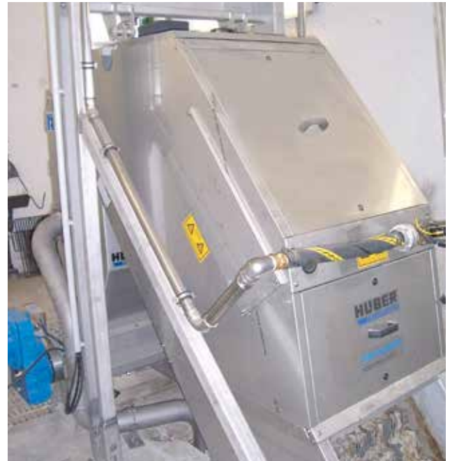
Fully enclosed, odour-free HUBER Fine Screen STEP SCREEN® SSF.
