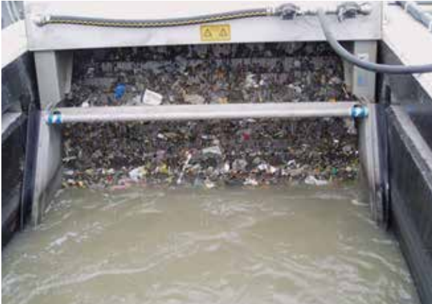
HUBER Fine Screen STEP SCREEN® SSF: length 3500 mm, width 1826 mm, 6 mm slot width, 50° installation angle. High capacity as the flow passes the screen surface only once.
