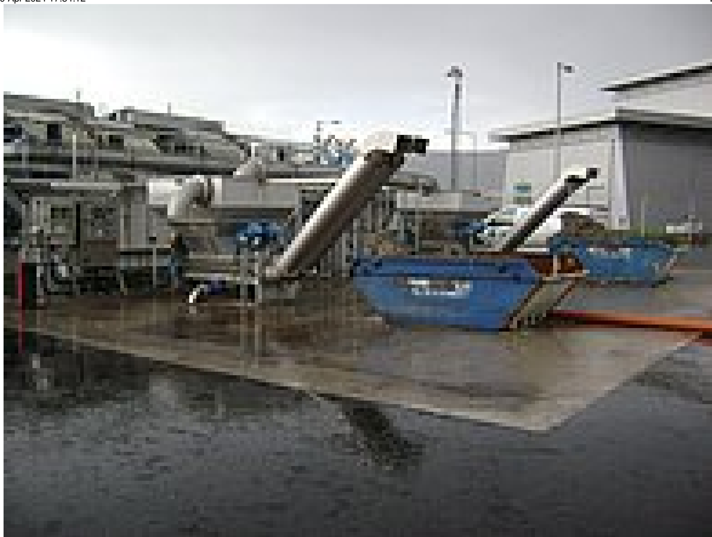
2 off HUBER Wash Press WAP-SL units designed for 15 m 3 /h raw screenings, via launder channel
